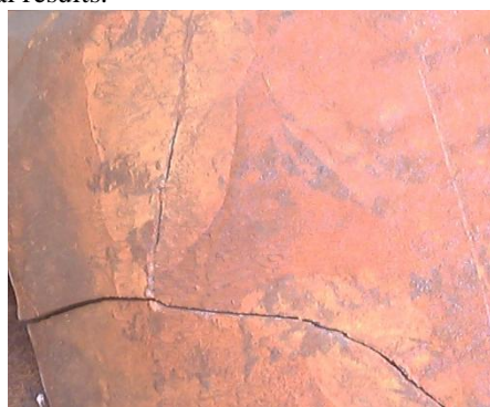
Fig 9. Cracks generated in the plate at edges
